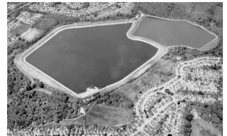
The picture below shows the adjacent reservoirs at Llanishen and Lisvane, which is the smaller of the two reservoirs.
