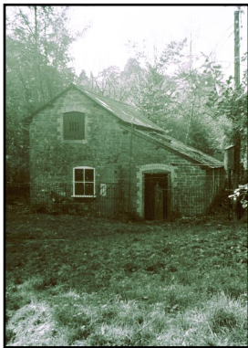
The pump house at Crooked Well (1973)
