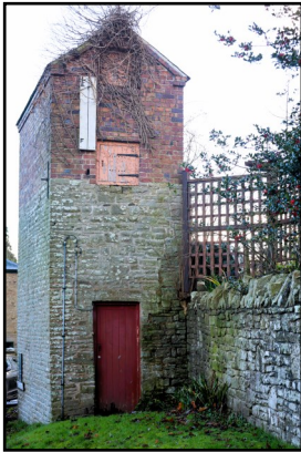
Kington Water Tower in January 2024
