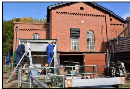
Oct 2020 Rolling shutter door being installed
