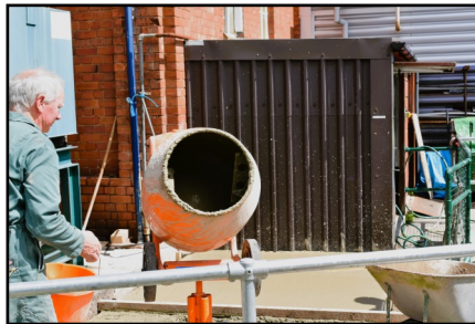
Sept 2018 Laying the display shed base
