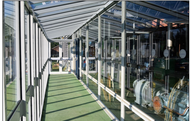
New elevated walkway and entrance to the Southall Gallery
